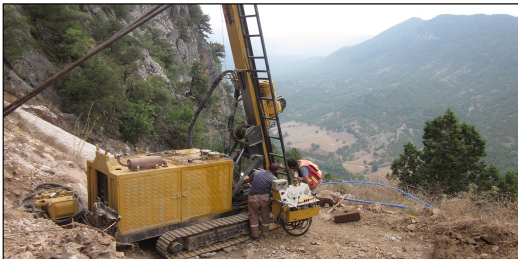
Figure 1: V004 drill Pad location & rig set-up at Pinargozu North. View towards the SSW.
